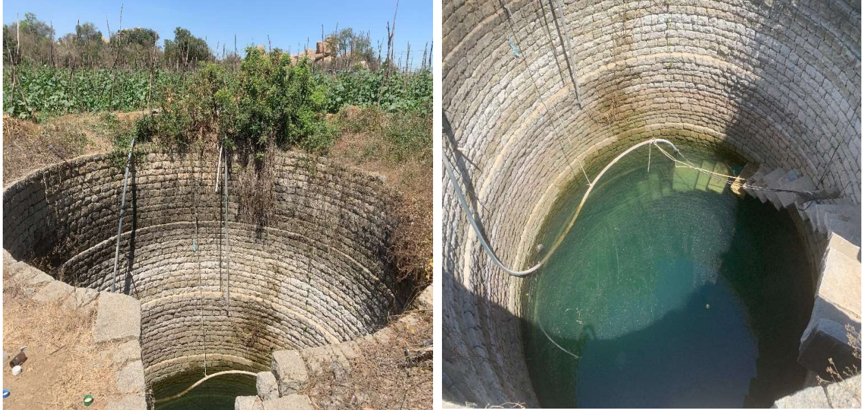
A traditional well with outer walls built using locally available granite stones is now equipped with an electric pump for water extraction.
