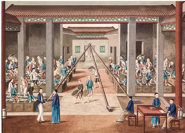
82. Tea Warehouse, 1820-1840, Guangzhou, China.
